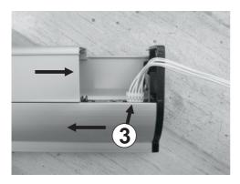
**3.** Connect the cable to the respective connector as shown in the picture. **4.** Refer to the installation manual to
